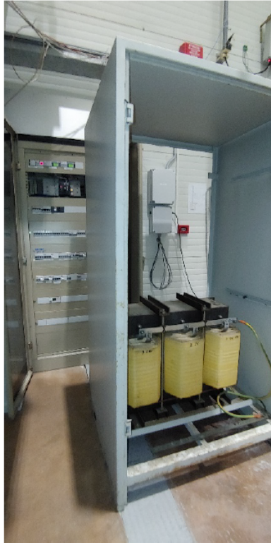
Fig.3: the available old insulation transformer used for the test
